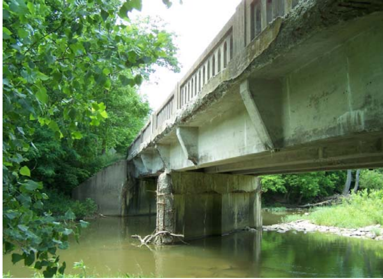
Exhibit 3: View of bridge substructure
