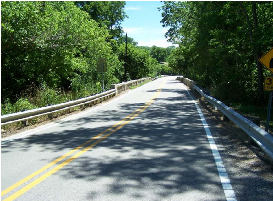
Exhibit 2: View of bridge and approaches
